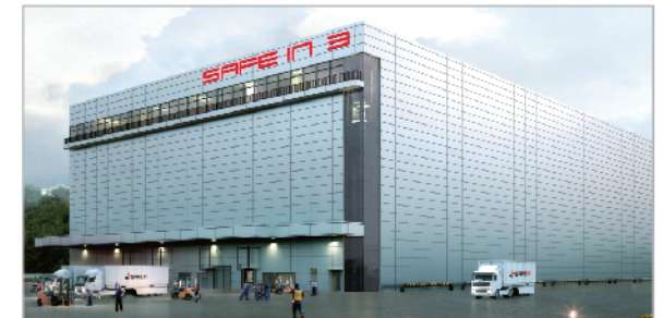
| 3rd. Automatic Storage Tower
